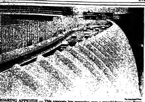
ROARING APPETITE — This concrete jaw swarming over a superhighway near Essen, West Germany, was erected to swallow the roar of the passing vehicles and protect nearby residents. The design of the anti-noise barrier is new and is reported to be highly efficient.
